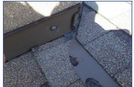
Section B - Deficiency #1 Improper installation of shingle step flashings
